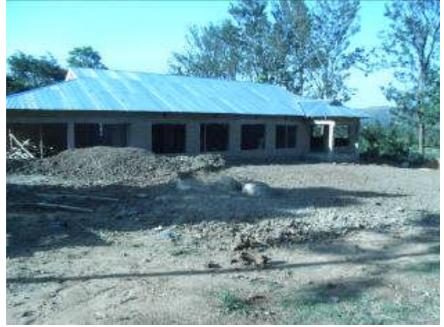
Second House in progress.
