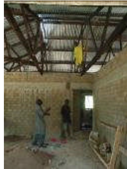
Electrical wiring going in
