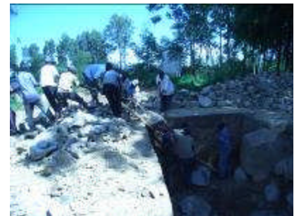
Digging through rock to create a septic tank.
