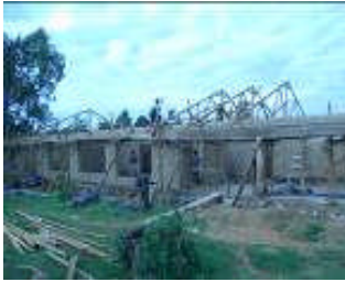
The trusses go up on house 1!
